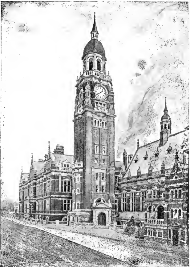
CROYDON TOWN HALL.
